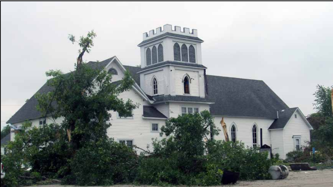
A severe storm that tore through Winger on Sunday night did extensive damage to several buildings, including Calvary Lutheran Church. The National Weather Service has not confirmed tornadic activity, though the damage seems to resemble that of a tornado.
