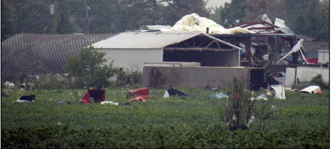
Buildings at Lucken Trucks and Parts in Winger had extensive damage along with debris strewn across the neighboring field after a severe storm passed through Winger late Sunday night.
