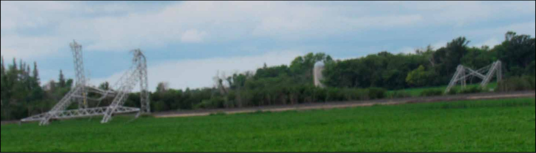
Electric power transmission lines from the Winger station to just south of Fosston were scattered and laying on the ground last Friday afternoon as high winds were a part of the dangerous storm that passed through East Polk County earlier that morning.
