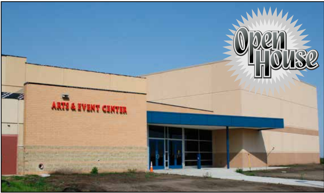
Nearly complete, the new Win-E-Mac Arts & Event Center will be ready for tours on Wednesday, September 2, 2015 during the open house from 5:00 pm to 7:00 pm.
