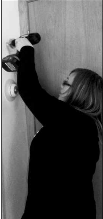
Good Samaritan Center employee Amy Rankin installing a CO detector.
