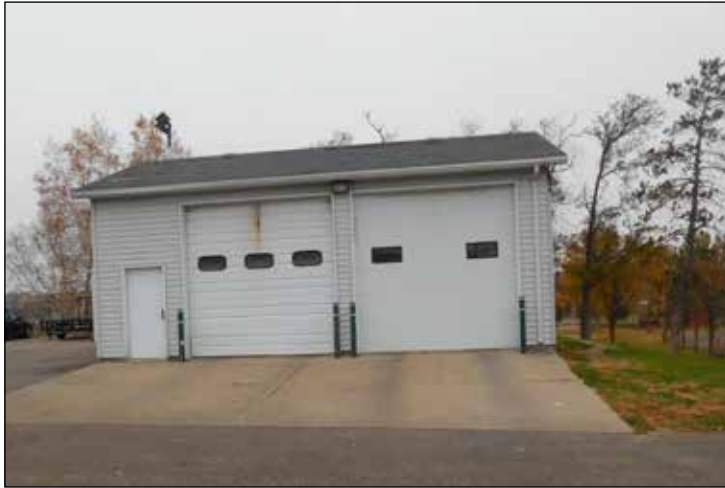
This 26 foot x 28 foot garage which previously housed the county ambulances will be moved by Randy Wettenkamp of Clearbrook. He submitted the only bid for the removal project. This will make room for the new helicopter pad by the hospital in Bagley.
