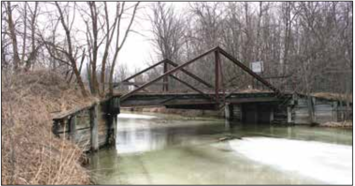
The bridge in Greenwood Township was built in 1905. It's a rare kingpost type bridge. One of two remaining in the state. This one is older than the other bridge (located near Luverne, MN) by about 3 years. The Luverne bridge is listed on the national registry of historic places.
