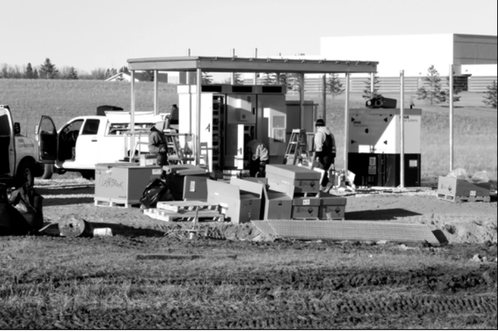
New tower "Going Up". There is a new Verizon cell tower being erected (near the school) on the north side of Clearbrook. This will improve Verizon cell service for the surrounding area. The tower should be in operation in a couple of weeks
