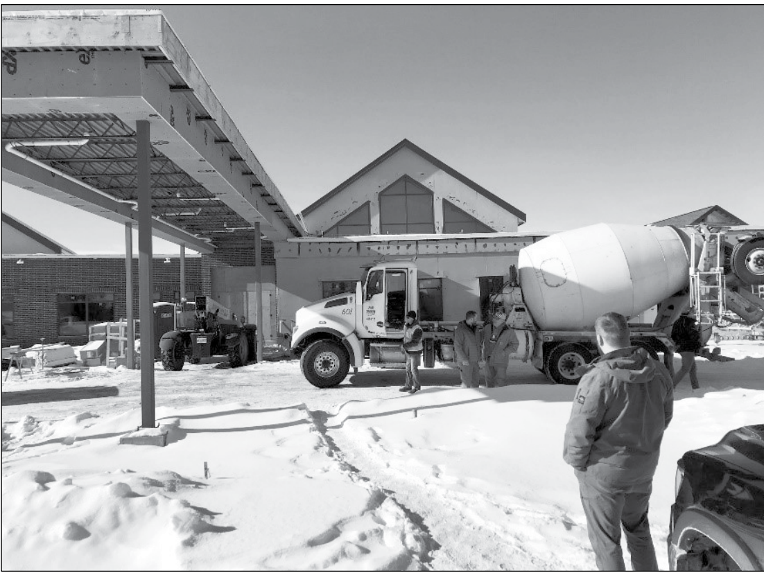
Pouring cement outside of the new Bemidji Veterans Home.
