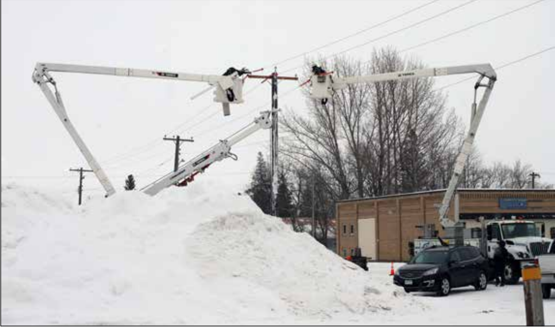
The light pole in Gonvick was hit and Ottertail Power Company and Gonvick Maintenance person Dan Johnson were able to put up a new one. Two trucks were able to make quick work of the setting of the new pole.
