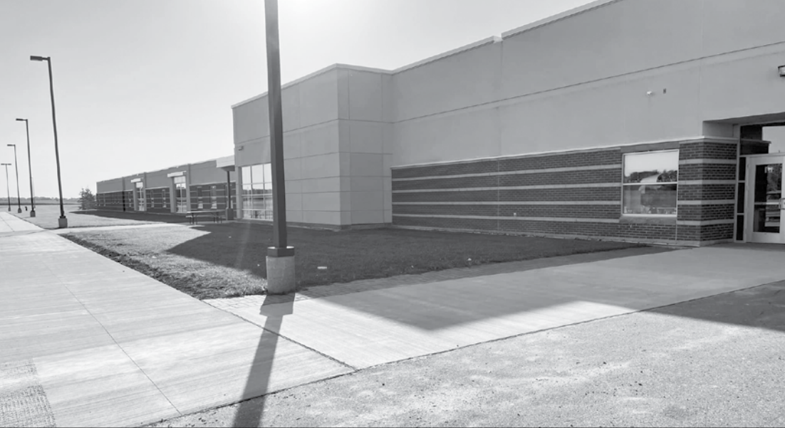
New sidewalk completed by Pond Construction on the north side of the school.
