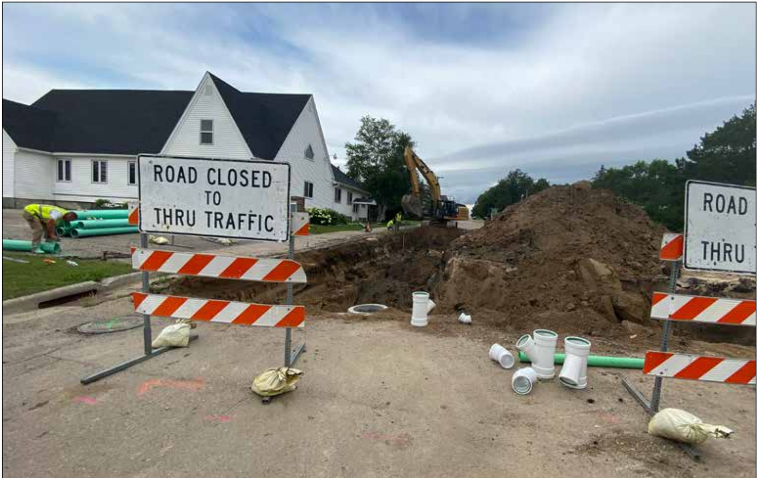
The water and sewer project in Clearbrook is progressing. Reiersen Construction has been working across Highway 92 on the west end of town digging and replacing pipes. When the pipe work is done on the east side they can start work on bringing the roads up to grade and get them ready for concrete. The concrete contractor should be coming up when that is done. There is lots to do on Hazel Ave and Jensen Ave.
