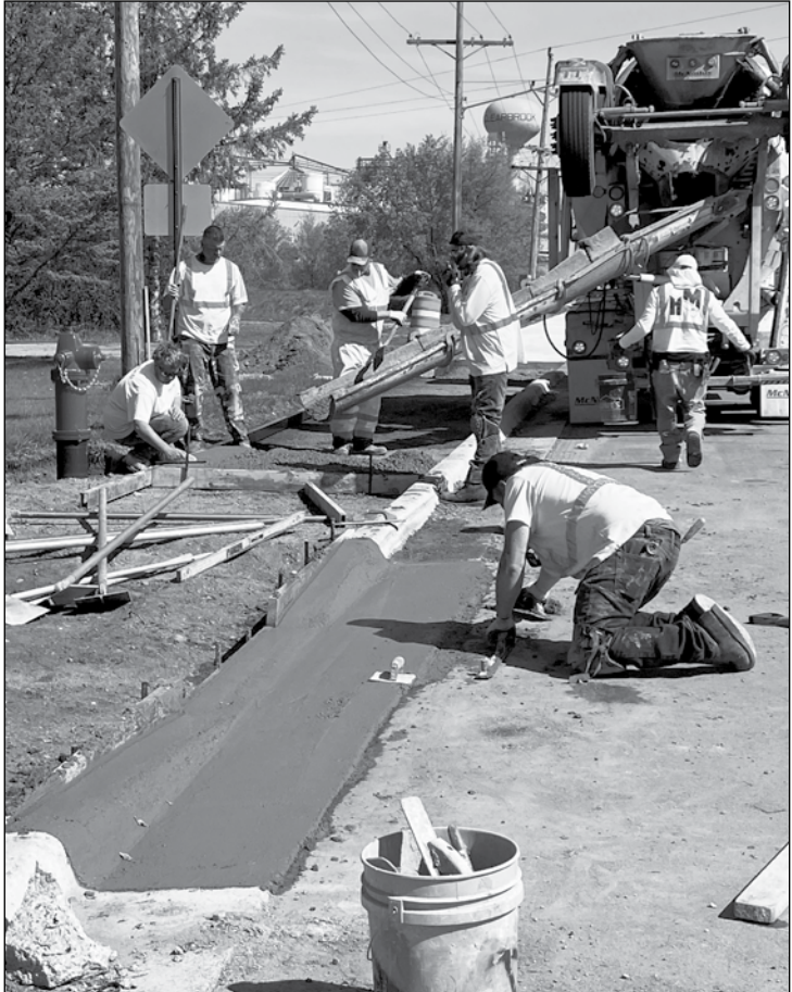
Curb and gutter going in for the Clearbrook street project.
