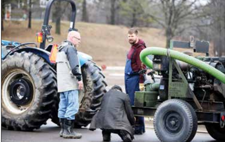
Clearbrook Mayor Dylan Goudge and Clearbrook Fire Chief Adam Krog looking at what to do to get water to go over Highway 5 between Y92 and Riviana Rice plant. The culvert was not allowing water to flow from the east side of the road fast enough.
