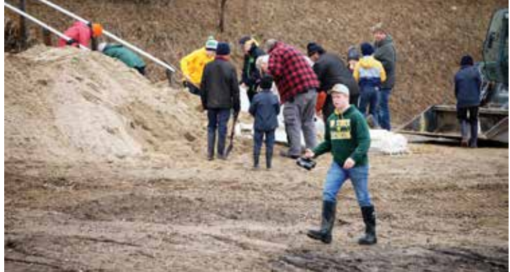
Workers were getting sand bags ready for the lift station in Clearbrook. The bags were put around and pumps were used to keep the equipment working.
