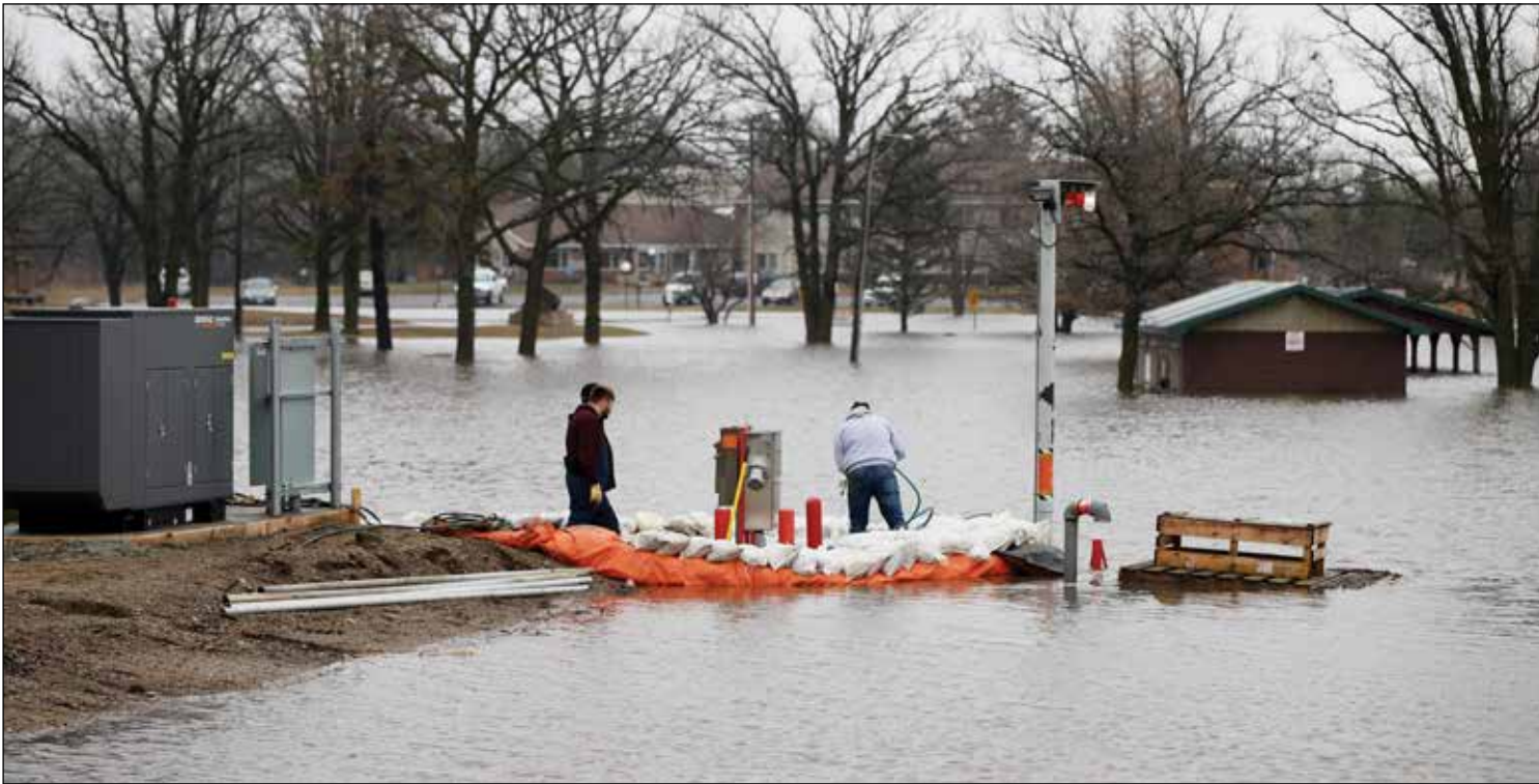
City of Clearbrook workers were busy at the lift station in Clearbrook. Sand bags were put around and pumps were used to keep the equipment working. Water was going up to the parking lot at Brookfield apartments. The picnic shelter is under water.
