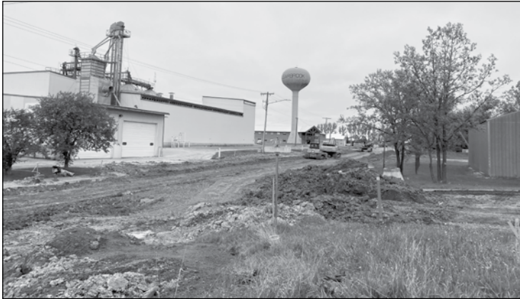
Sewer and water project in Clearbrook.
