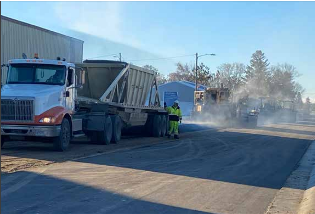
Some roads in Clearbrook are getting tar this week. This photo is from the north heading south towards the old school on the east side. The road north of Y92 and Northdale has one coat and eventually there will be three coats put on.
