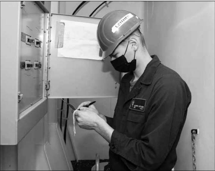
SAN DIEGO (Sept. 29, 2021) Damage Controlman Fireman Joseph Leitner, from Bemidji, Minnesota, hangs a safety tag on a breaker while performing maintenance on a fuse panel aboard amphibious assault ship USS Tripoli (LHA 7). Tripoli is an America-class amphibious assault ship homeported in San Diego. (U.S. Navy photo by Mass Communication Specialist Seaman Maci Sternod)
