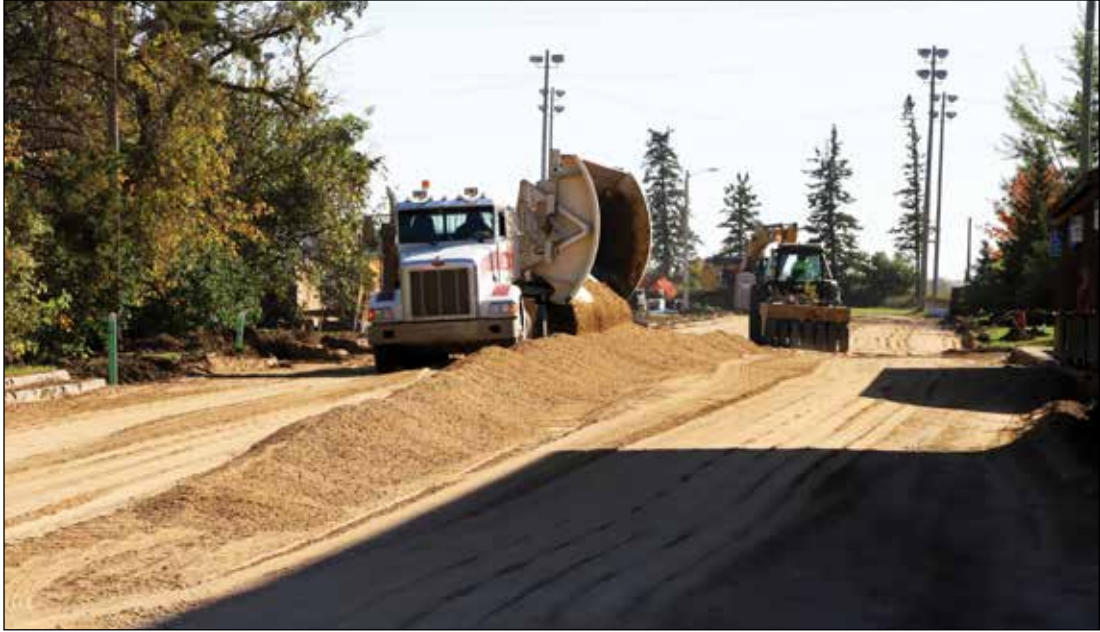
Getting ready for tar on some streets in Clearbrook before winter sets in.
