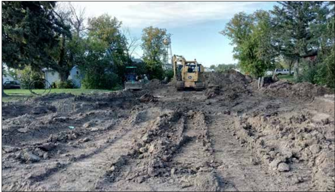
Construction on the streets in Clearbrook is still a long way from done. Some of the streets were to be tarred before winter sets in.
