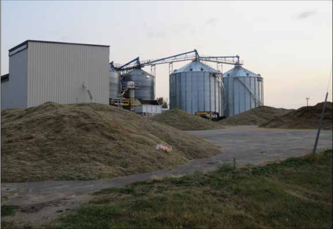
Wild rice is coming in to Riviana plant in Clearbrook for processing.
