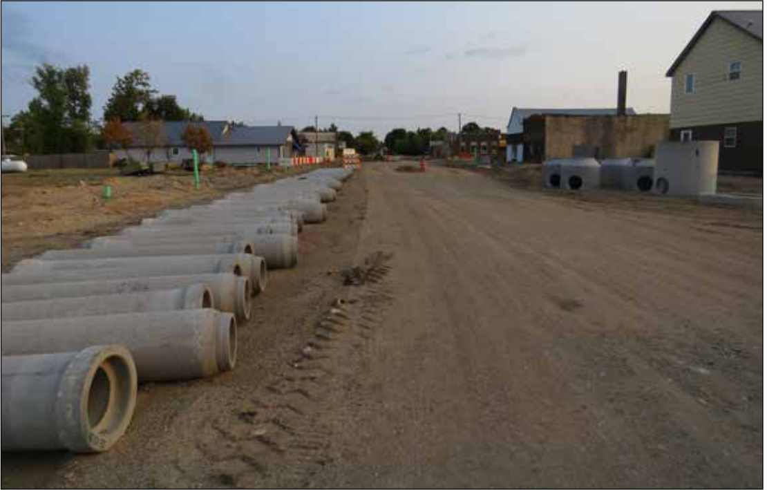
Construction on the roads in Clearbrook has been moving along. This shows what is left to be done on Main Street in Clearbrook.
