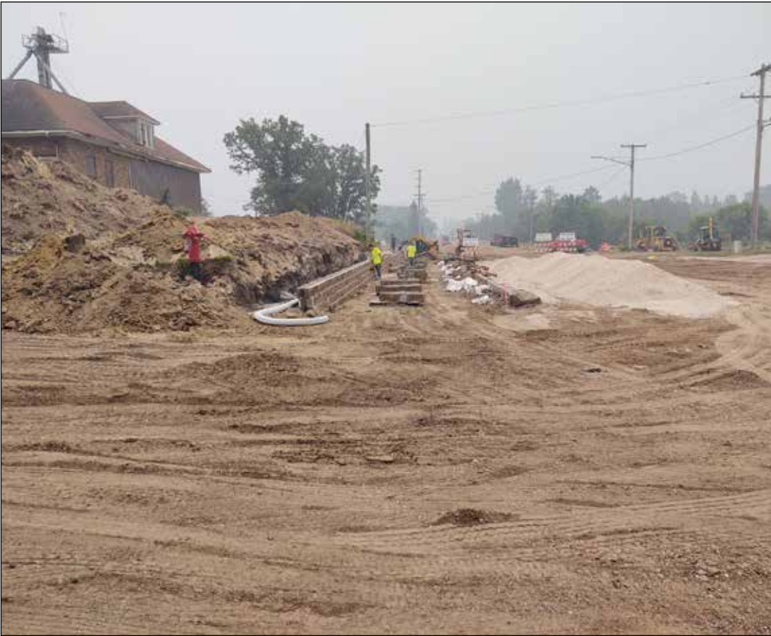
Check out the progress on the Clearbrook Bike Trail. The contractor is installing the new retaining wall.
