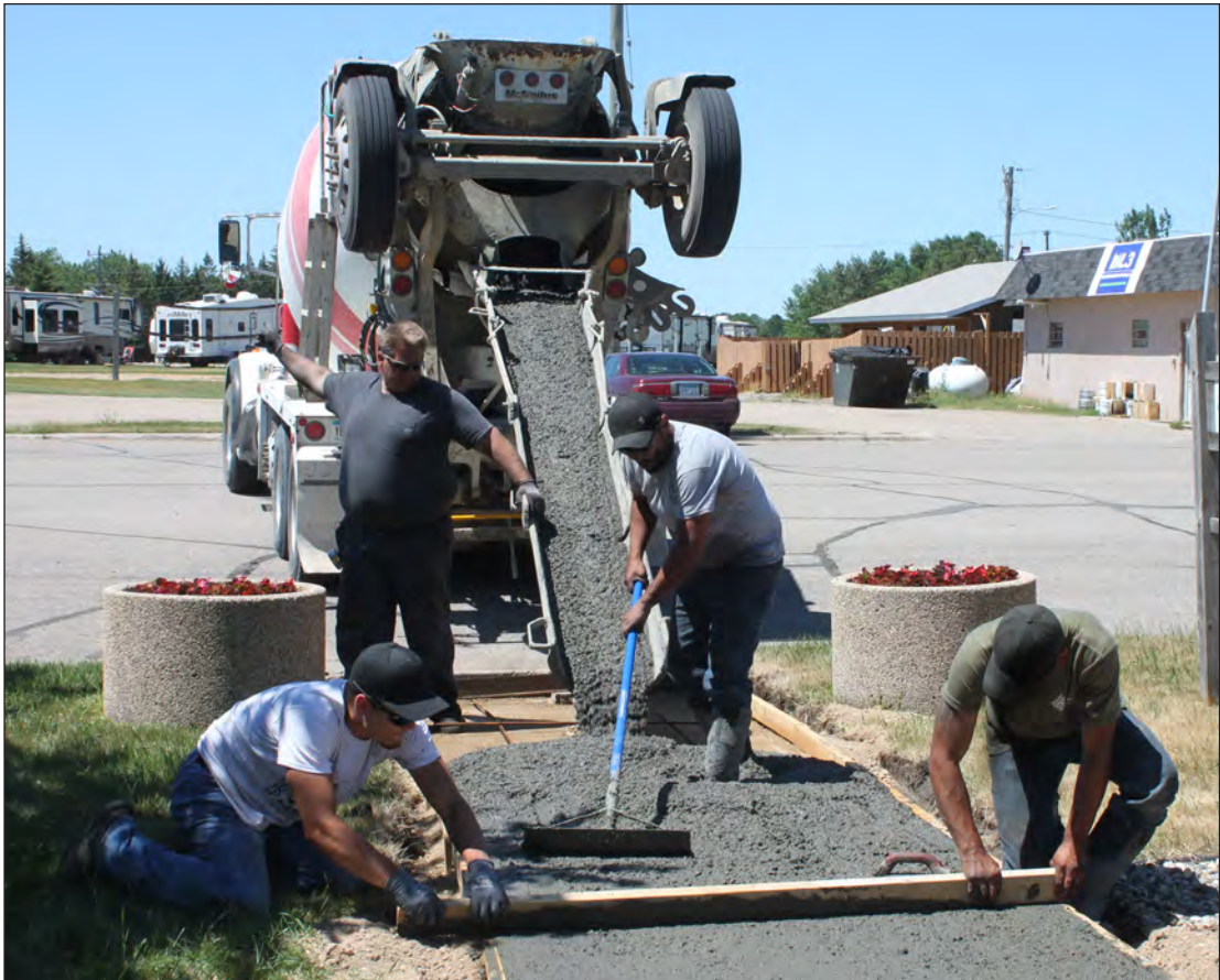
New sidewalks are being poured in preparation for the All-School Reunion in Gonvick set for July 8, 9, 10 and 11. Gustafson and Goudge workers were busy with Paul Nelson directing the flow of the cement. The walks were being replaced by the Gonvick Community Center.
