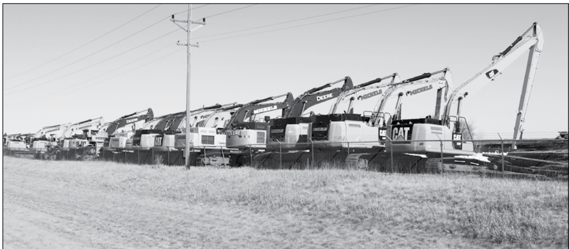
Equipment has been shut down temporarily for Line 3 for a couple of days due to some road restrictions. They will be starting up again as soon as the spring road is back in shape.
