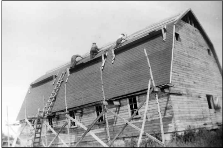
A barn building crew at work in 1949.
