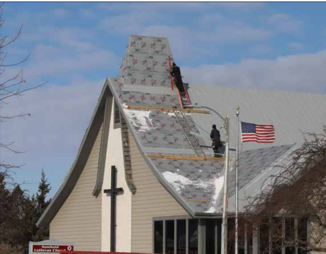
New roofing material going on the Samhold Lutheran Church in Gonvick.
