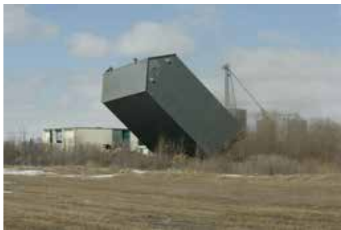
Sun Plant building going down.
