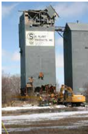
Getting ready to take down the Sun Plnt in Gonvick.
