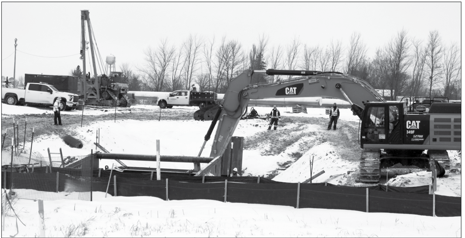
Pipeline work in Clearbrook is going on strong this week. This picture was taken on the south side of Clearbrook. You can see the old watertower in the background.
