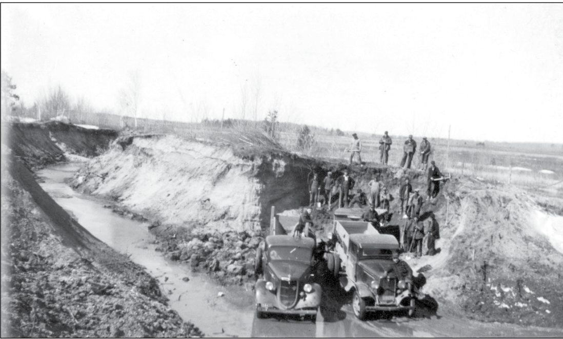
A road project.
