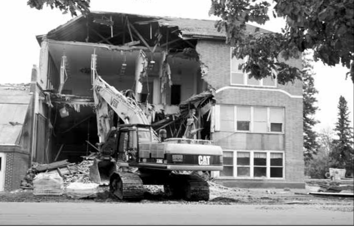
End of an era.. Gonvick School building torn down.
