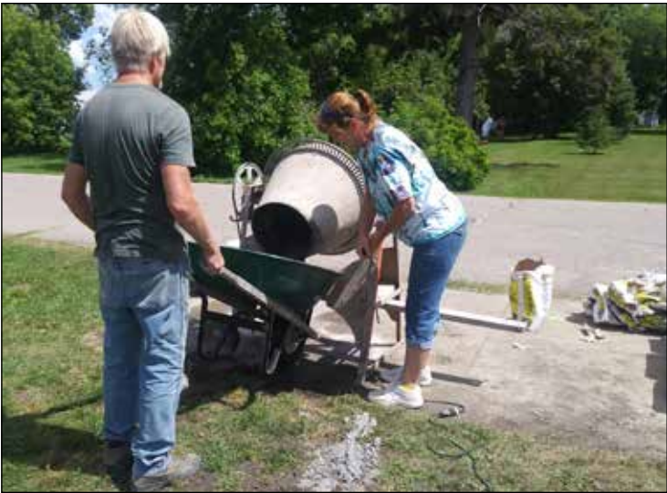
Randy Helgeson & Kimberley Nelson mixing cement.
