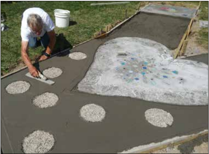
Bruce Brunsberg smoothing out the concrete.
