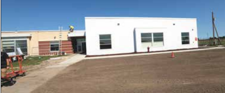
The new portion of the school was extended as far as the fire hydrant to the south of the building. The grounds around the building was still being prepared.
