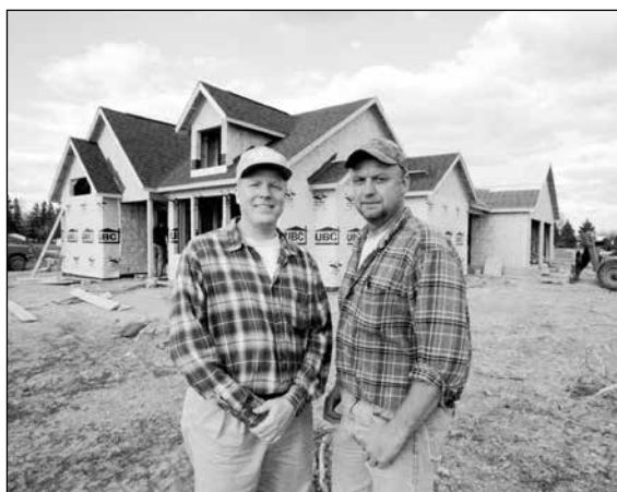
James Scott Enterprise LLC new house being built on the SW corner of the old Football field. Shown are Jim Clemenson and Scott Fawver.
