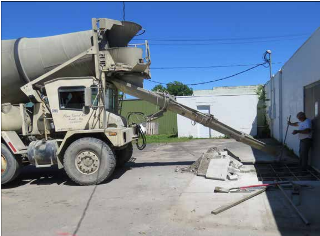
Cement poured in Gonvick by Olson Gravel Inc from Trail.
