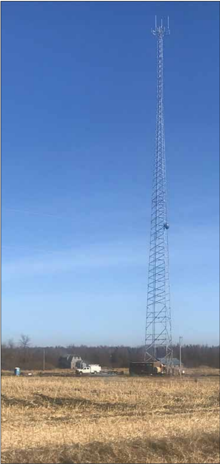
New tower goes up east of Berner.
