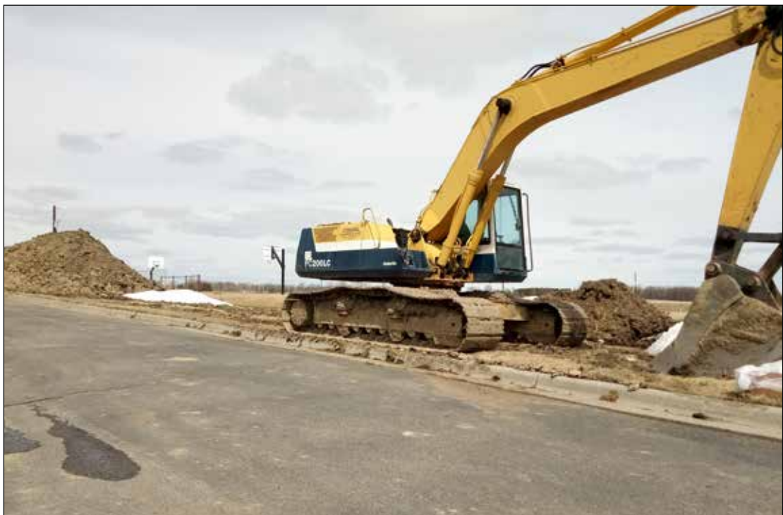
Dyrdahl Construction with their equipment at the Clearbrook-Gonvick School.
