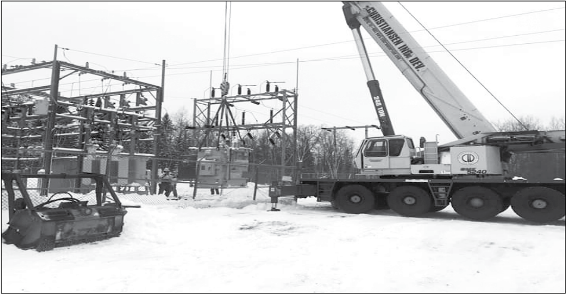
The Dudley Substation had an outage on Saturday, Minnkota crews had to come in an install a new transformer. It was a 40,000 pound 2,500 transformer along with the crane and crew from Minnkota. People in that area were without power until 5:00 that afternoon.
