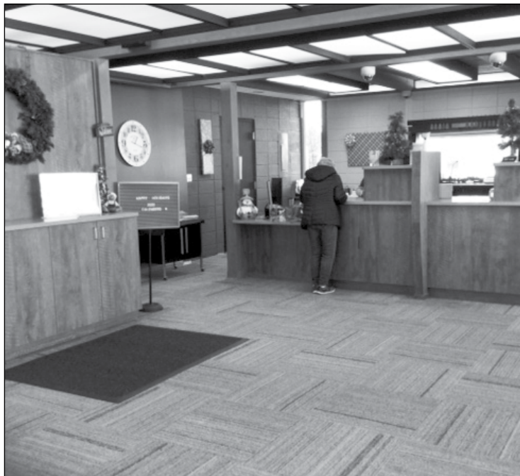
After months of work, the remodeling has been transforming. The lobby is larger and the teller stations are more functional. Photo by Security State Bank.
