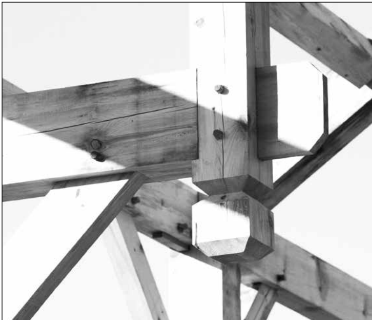
This view shows how some of the pieces tie together in the frame. Note the mortise and tenon join in the center of the photo, with handmade white oak pegs to keep the pieces secured. Other such joints don’t go all the way through the beams.
