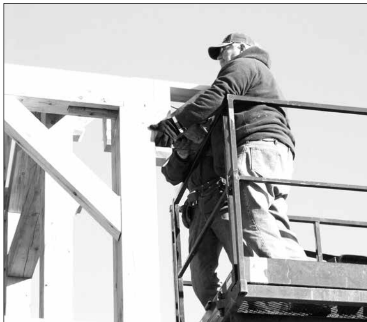
Jon Bachmann (foreground) holds a pre-assembled brace in place while John Sandland screws it into place.
