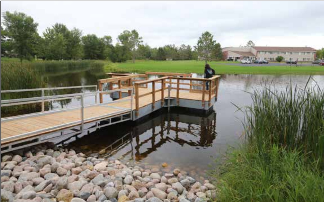
The fishing pier was built by MN Boardwalks, LLC of Glencoe, Minnesota. It was designed to remain in the water all year. Many visitors to the pond have already found success while fishing from the pier. The Minnesota DNR has supported the project by stocking the pond with a variety of fish, including crappies, bluegills, and bass.
