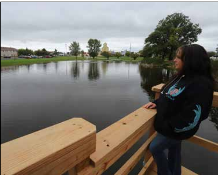
Laura Grant is pictured here, enjoying the view from the new fishing pier at the Clearbrook Pond. The pier was funded by a $15,500 grant from the TEAM Industries Foundation and is one of the latest improvements being made to the Clearbrook dam area.
