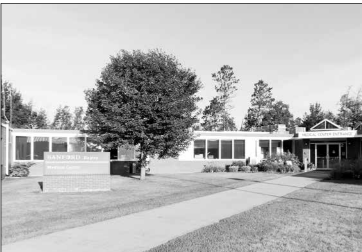
Sanford hospital improvements include HVAC ducting seen on the top of the building for air-conditioning and heating. Rob says this is not completely efficient, but is a great improvement in the heating and cooling of the patient and other rooms, and less costly.
