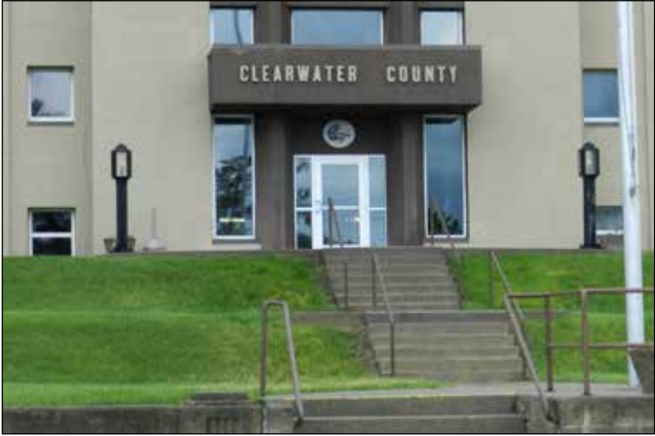
A new front door was recently installed at the Courthouse.
