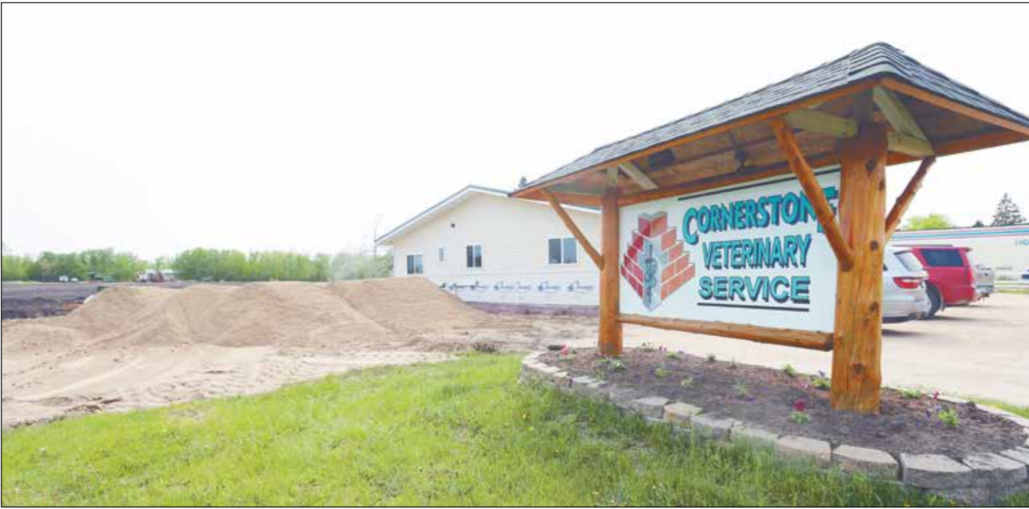
The question was what is all the dirt for? Cornerstone Veterinary Service is adding on to their facilities in Gonvick. People will be able to bring their larger animals instead of the service going out to the farms.
