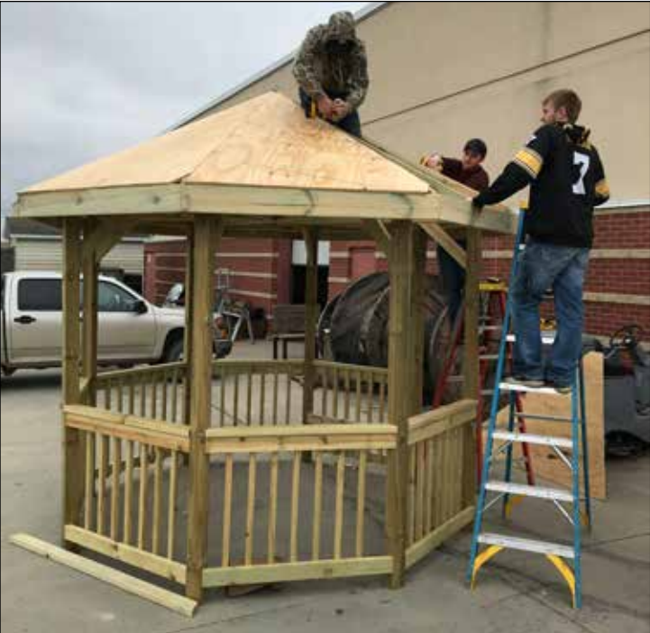
Students Brandon Quern, Erick Bergman, and Levi Nelson installing roof sheathing on the gazebo being built by Clearbrook-Gonvick shop students.
