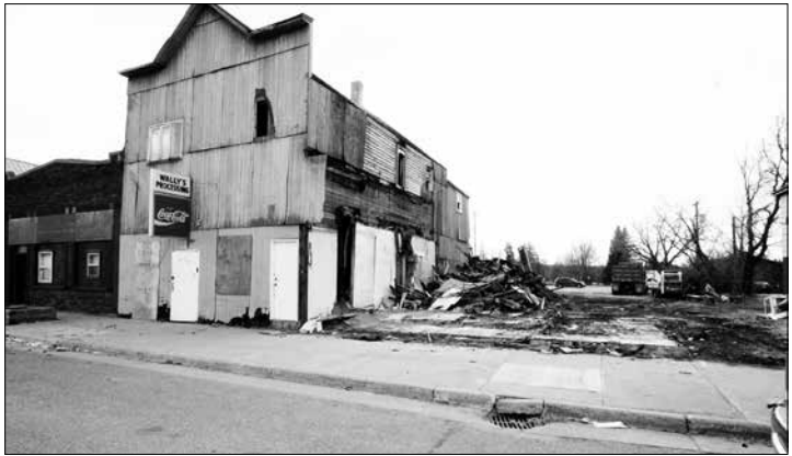
Jorgenson Backhoe and Consturction has half the building down. What is left is the original building before the addition was added.
