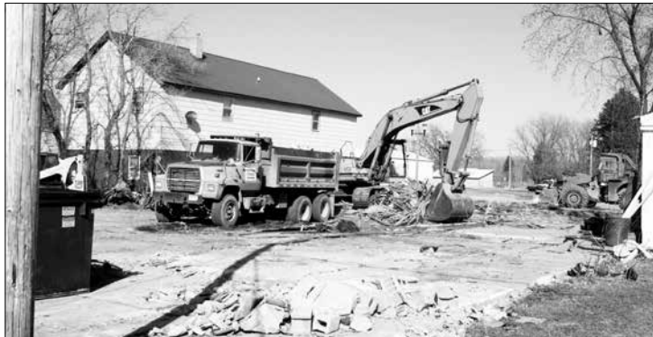
The last of the clean-up of the 1910 building from Main Street in Clearbrook. Jeff, who is the owner of Jorgenson Backhoe & Construction works with business and industry in the construction trade in a wide area.
