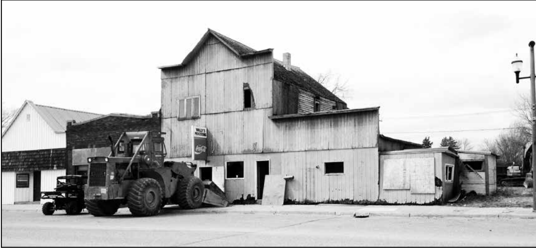
Getting ready to take the old building down on Main Street in Clearbrook.
