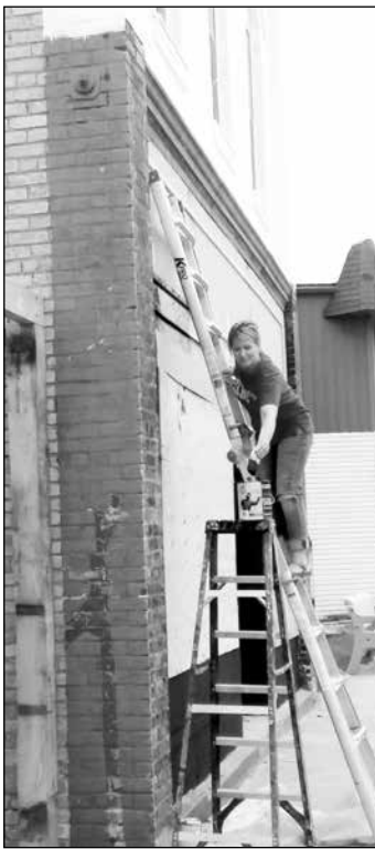
Andrea Stordahl painting the outside of the building.
