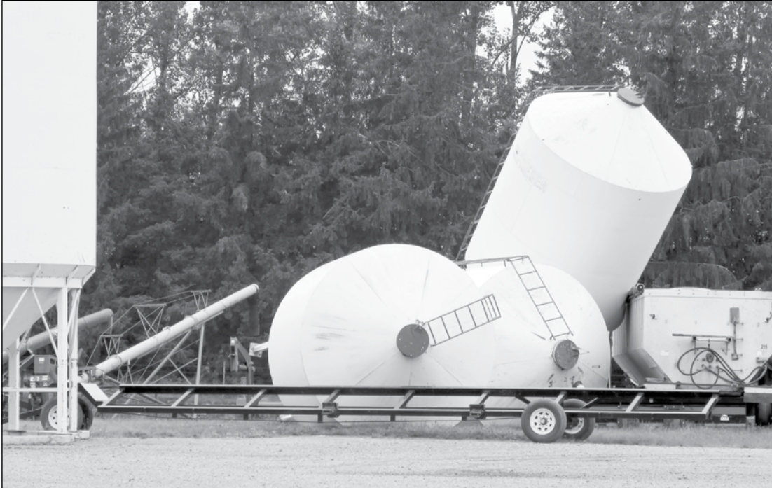
Tanks tipped over after the storm on Monday morning.
