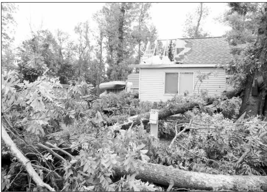
The roof of one of Charps buildings in Clearbrook was peeled back and some blown off. The white stuff all over the ground and on the green part of the building was installation. Most of the roof was cross the road in the soy bean field.
