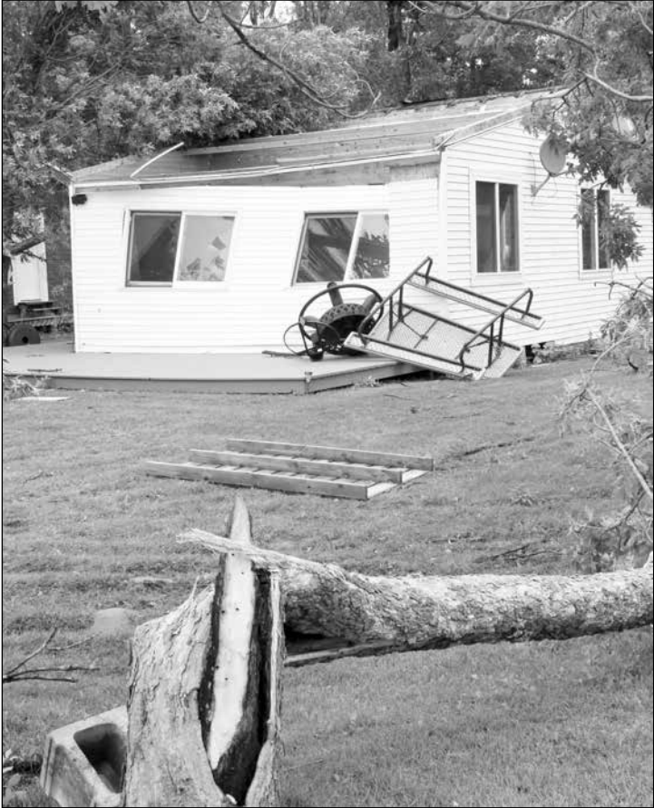
Pete and Becky Erickson from Warren had considerable damage to their cabin on Pine Lake.
