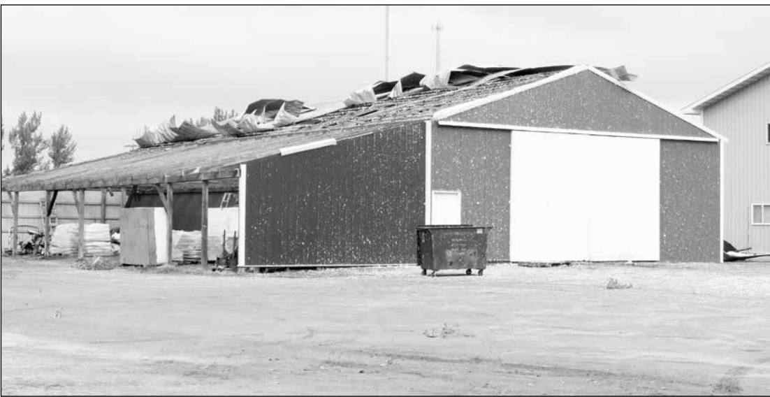
The roof of one of Charps buildings in Clearbrook was peeled back and some blown off. The white stuff all over the ground and on the green part of the building was installation. Most of the roof was cross the road in the soy bean field.
