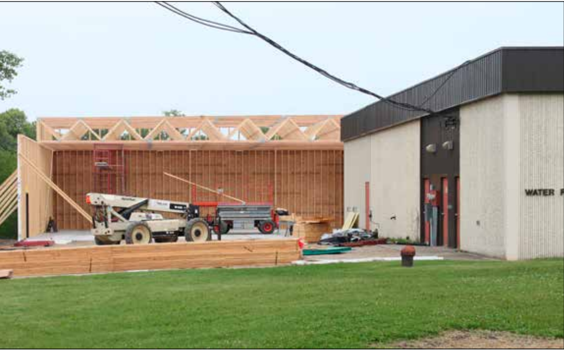
The John and Faye Hedin addition in progress at the Gonvick Fire Department.
