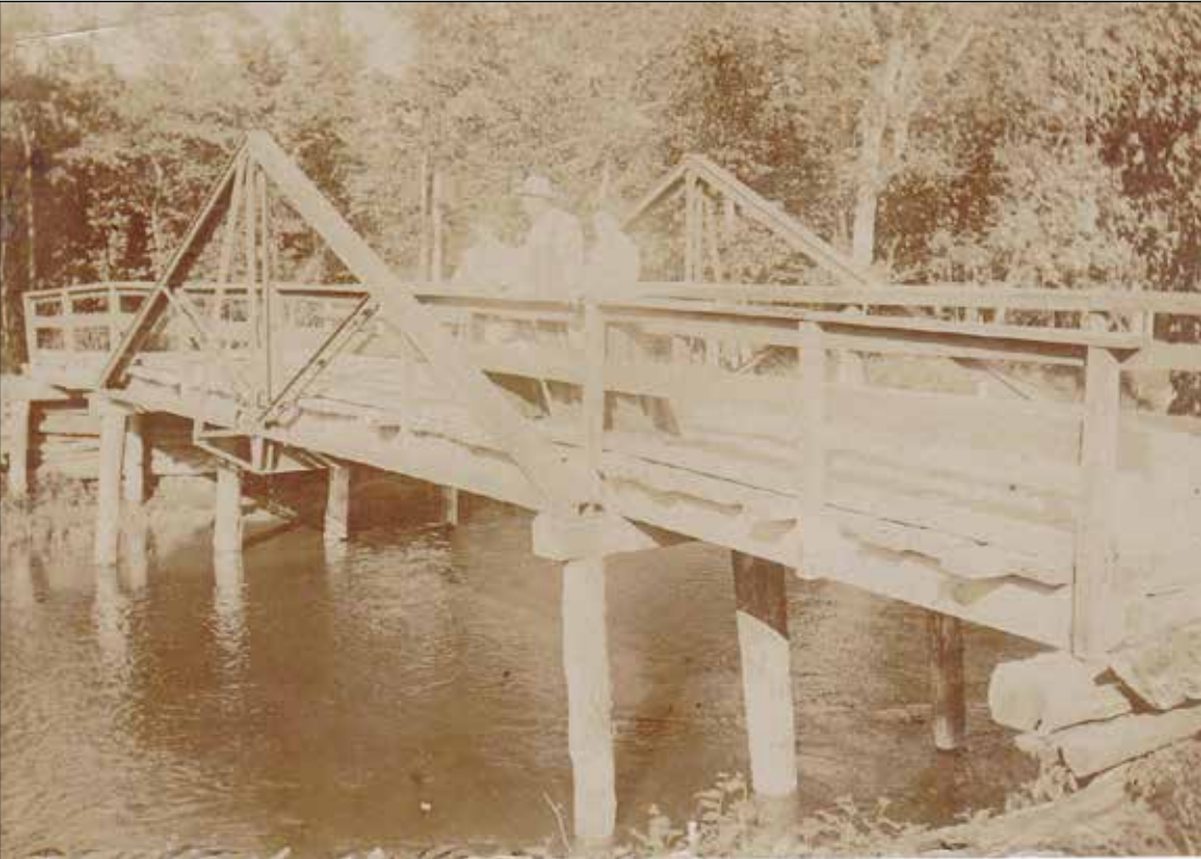
The Greenwood Bridge was built in 1905 and this pictures was taken in the early 1900's The king post truss is used for simple roof trusses and short-span bridges.
