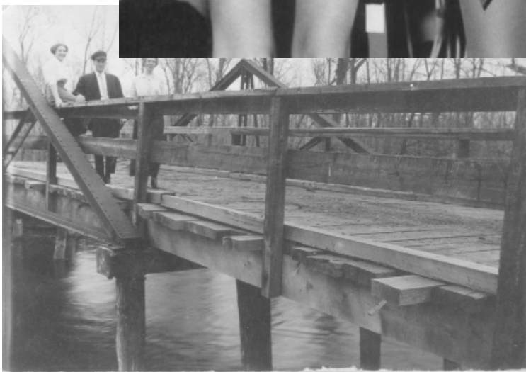
November is Historic Bridge Awareness Month. This is a King Post Truss number L1297. It was constructed in 1905 over the Clearwater River in Gre Township. It was moved to the Lake Itasca Pioneer Farmers Show grounds a fe ago. The first photo was taken in 1913. The second, just before it was moved i
