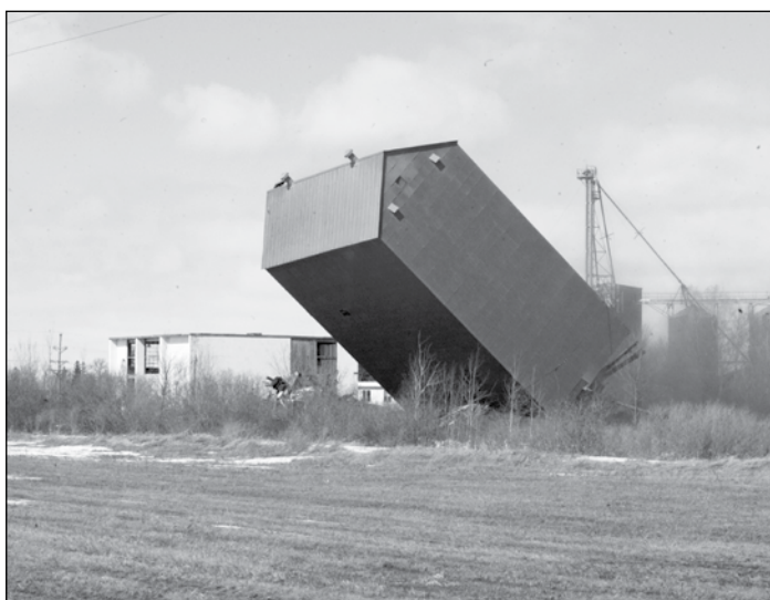
Getting ready to take down the Sun Plant in Gonvick.
