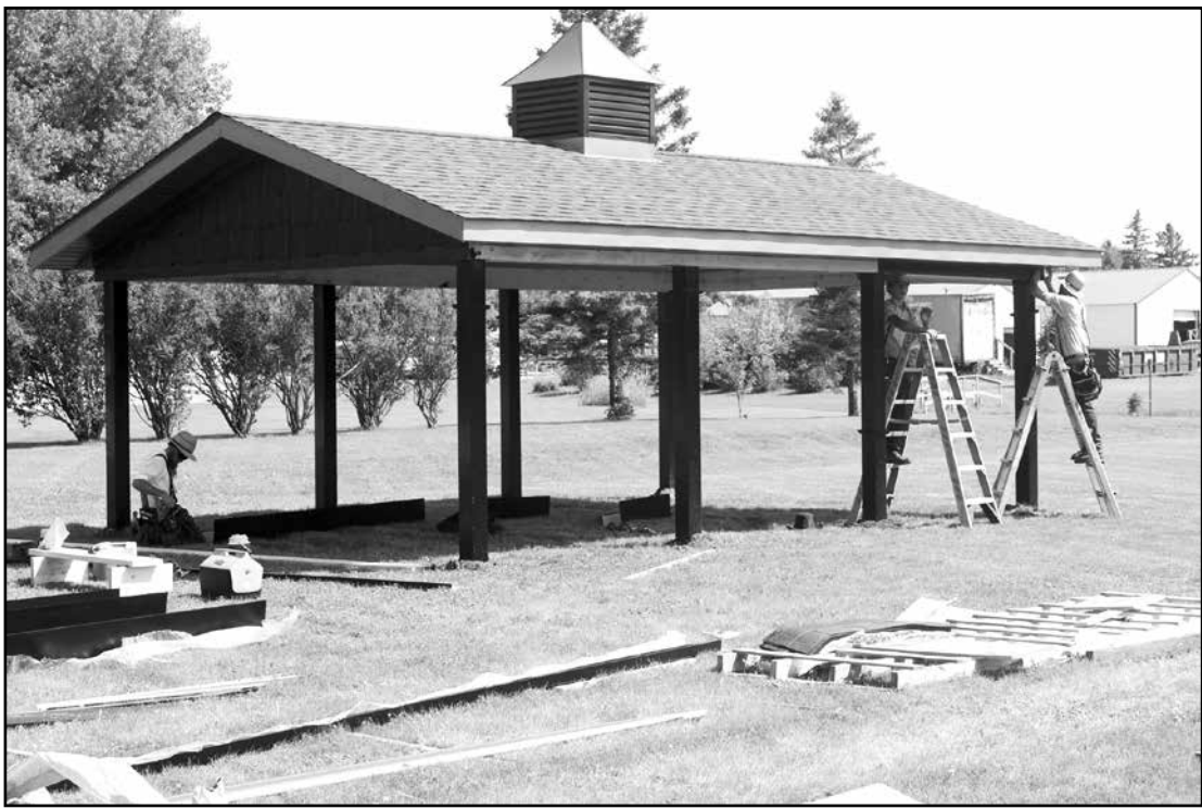
Check out the new picnic shelter at the Goodridge Veteran's Memorial Park. Dan Mast & crew of Mast Home Improvement completed the work and finished adding the iron railing with granite plaques. The shelter is made possible with a $750 grant from Operation Round-Up of Red Lake Cooperative and also from various fundraisers around the Goodridge Community. Plans for the shelter will include the placement of centennial picnic tables that were designated to stay in the park.
