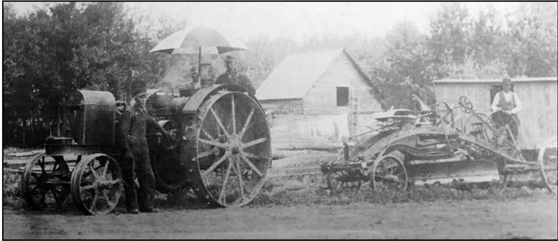
Grading on Hwy 89 through Grygla in 1910. Fladland's barn is in the background. The location is west of the Coop Store. Otto Lee is operating the grader, his son, Henry Lee, is on the tractor and a Mr. Lund is also pictured.
