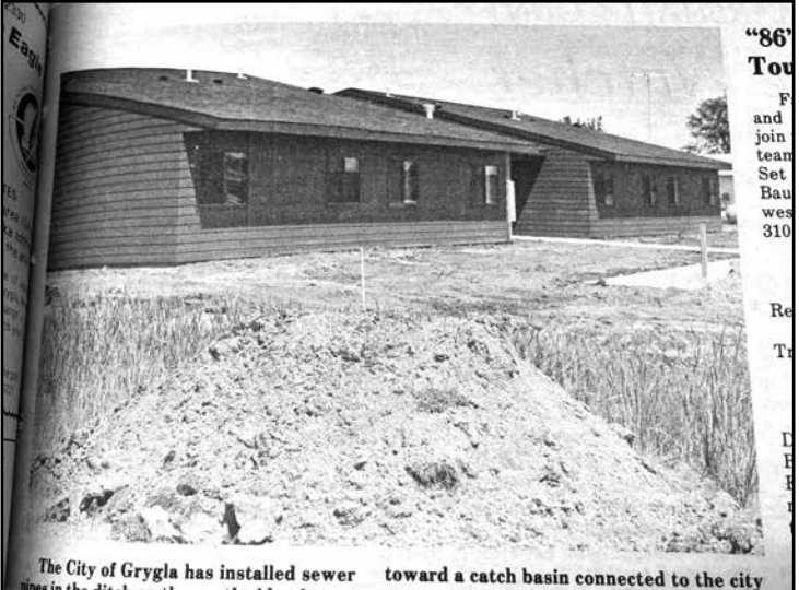
The City of Grygla has installed sewer pipes in the ditch on the south side of town which is normally filled with standing water and cattails. They are now in the process of filling the ditch and sloping it toward a catch basin connected to the city storm sewer. In the background here is the new 8 unit MarBell Homes apartment building which was completed this spring.
