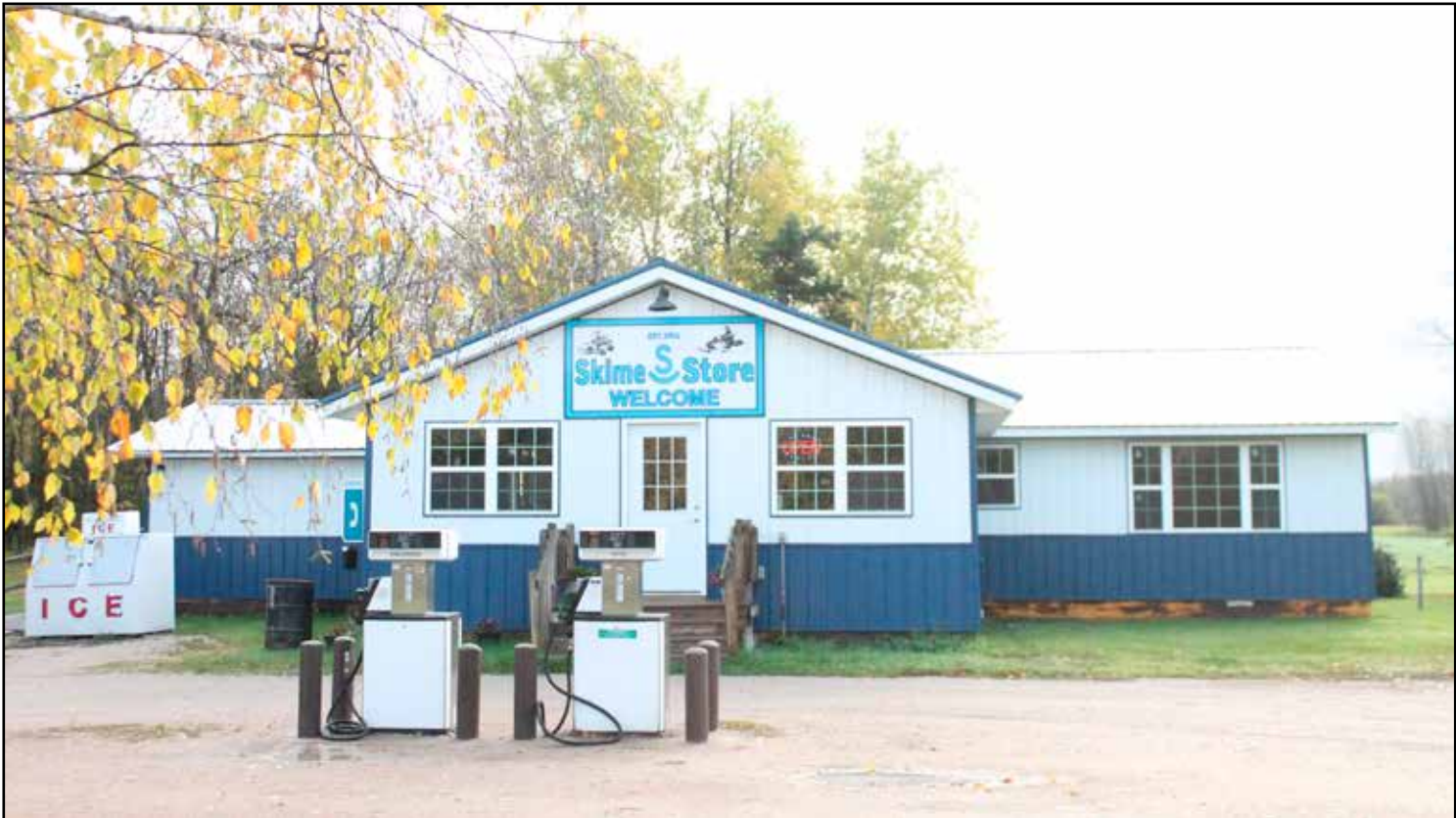
With new white and blue tin, the Skime Store closely resembles its past version. Along with new siding, the store also got new windows, a new roof and some updates inside. Photo by Grygla Eagle Newspaper
